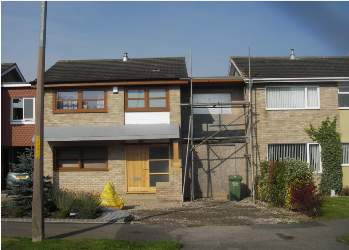
b) Rear elevation of application site as of 3 rd October 2011
